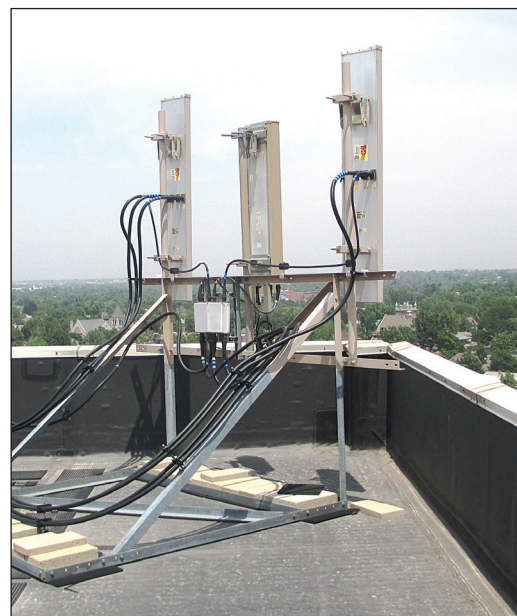
Figure 1. Rooftop antenna installation
